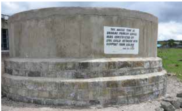
Primary School Water Tank, Kenya. Source: Aidlink
